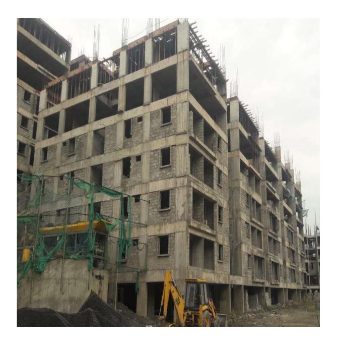
**Block D1:** Shuttering & Barbending works for 2<sup>nd</sup> half of Seventh Floor level slab 30% completed and balance works on progress. Columns upto 8<sup>th</sup> floor level 45% completed
