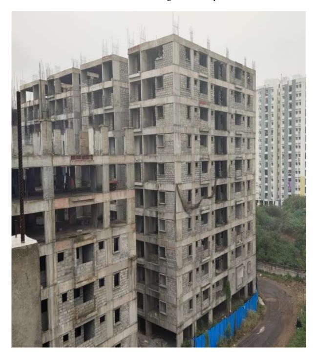
**Block D3:** Ninth Floor level slab 1<sup>st</sup> Half Concrete casting 100% completed and balance works on progress.
