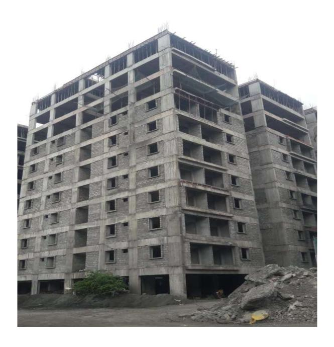
**Block C3:** Shuttering works for 2<sup>nd</sup> half of Seventh floor level slab 60% completed and balance works on progress.
