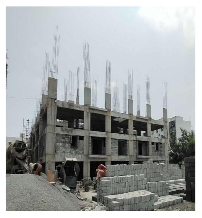
**Block C1:** Terrace Floor level slab concrete 100% completed.
